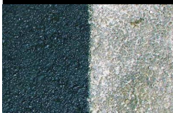
After Seal Coating Before Seal Coating
