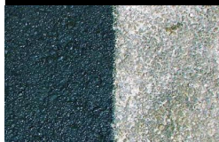
After Seal Coating Before Seal Coating
