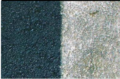
After Seal Coating Before Seal Coating
